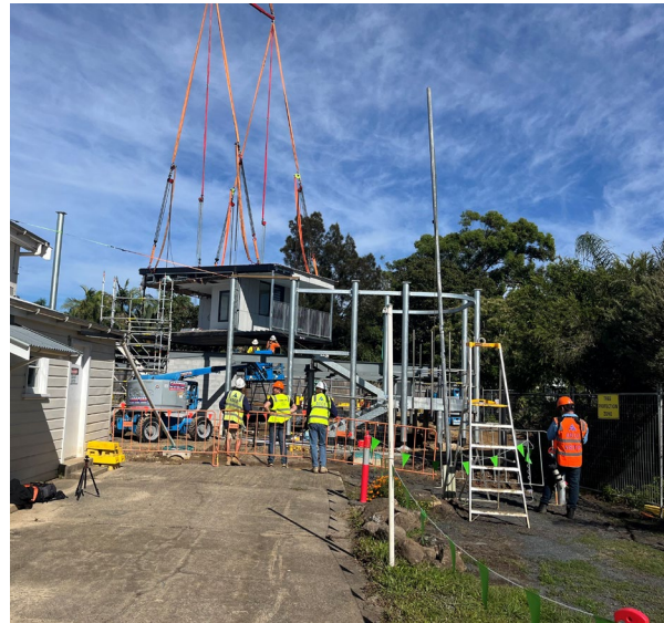
Volumetric Construction, Flood Recovery Schools, NSW Northern Rivers
