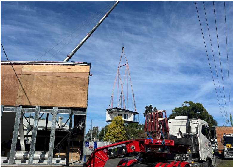
Volumetric Construction, Flood Recovery Schools, NSW Northern Rivers
